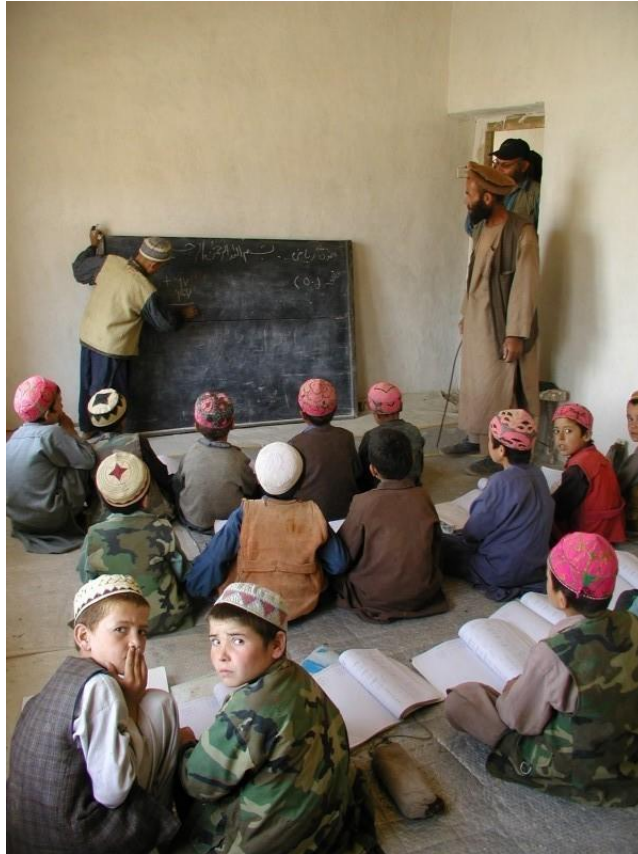
Dasht e Freng village primary school, Shahr-i-Buzurg district of Badakhshan province, Afghanistan, constructed by Oxfam GB in 2002 (Photo: Yasin/Oxfam)
